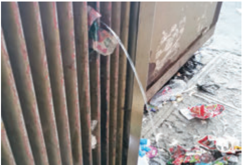
Transformer oil draining from a vandalised mini-substation’s transformer.
